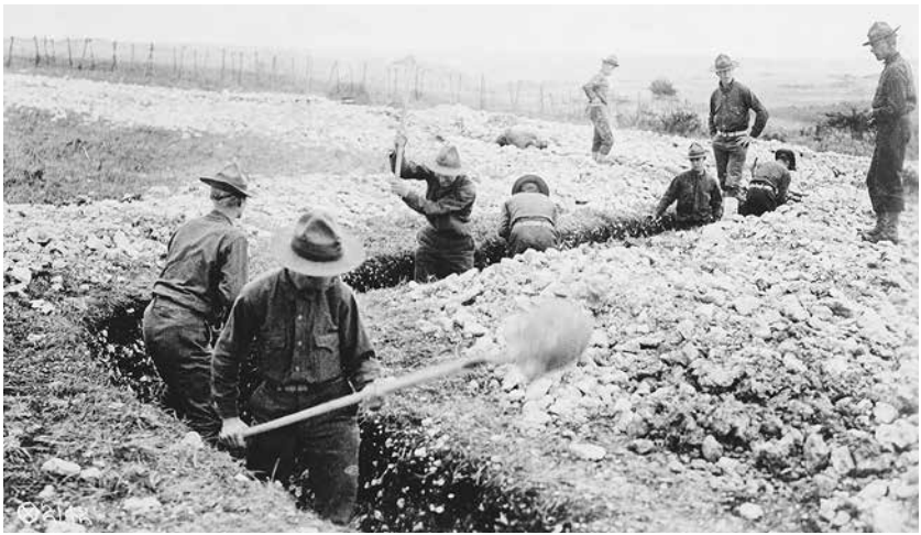
Building a mock trench system (Library of Congress)
